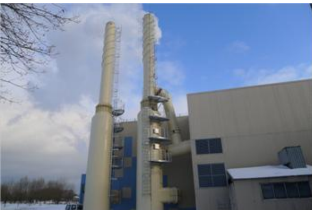
Flue gas condensers saving 10-15% of wood fuel
